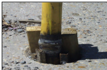
Figure 2. Post at intersection of Route 155 and Route 249.
