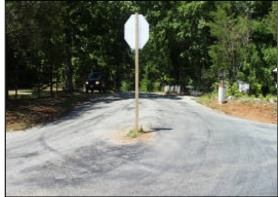
Figure 16. Intersection of Route 615 and Route 628.
