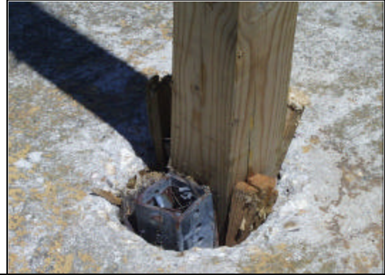
Figure 14. Sign post at the intersection of Route 605 and Route 622.
