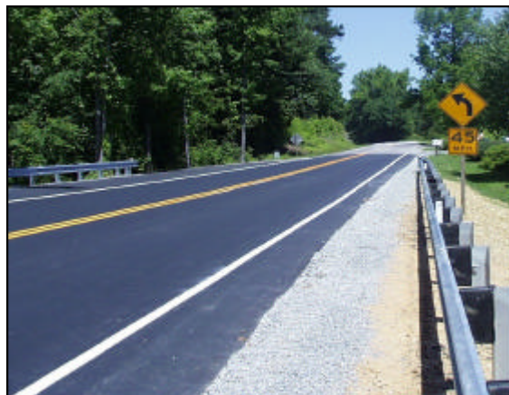
Figure 11. Maximum safe speed in curve sign, Route 5.
