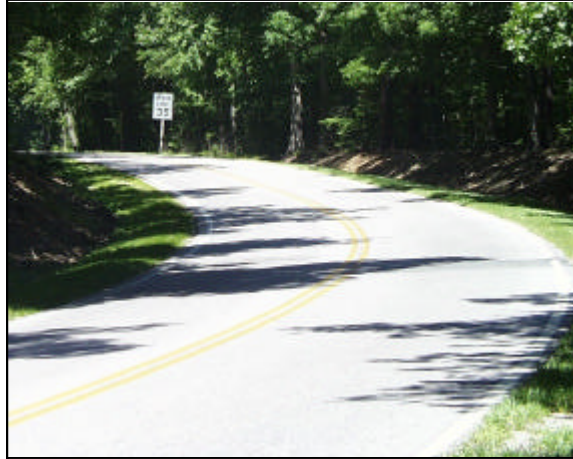
Figure 10. Curve on Route 5.
