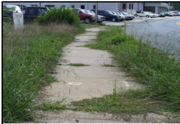
Figure 2: Sidewalk with overgrown vegetation.
