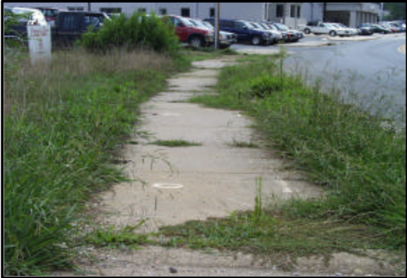
Figure 2: Sidewalk with overgrown vegetation.
