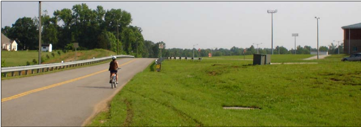
Figure 4: Bulldog Way (Route 724) was built in 2004. Goochland High School is on the right.
