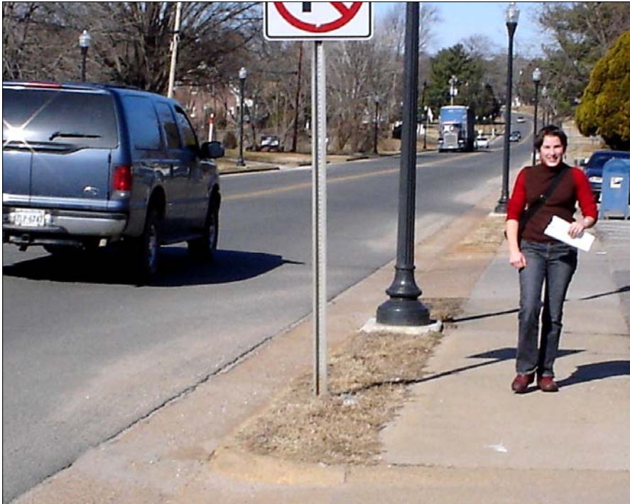
Figure 2: River Road West (Route 522/6) in central courthouse area, looking north. Note the wide outside lane, frequent curb cuts, streetlights, and sidewalks.
