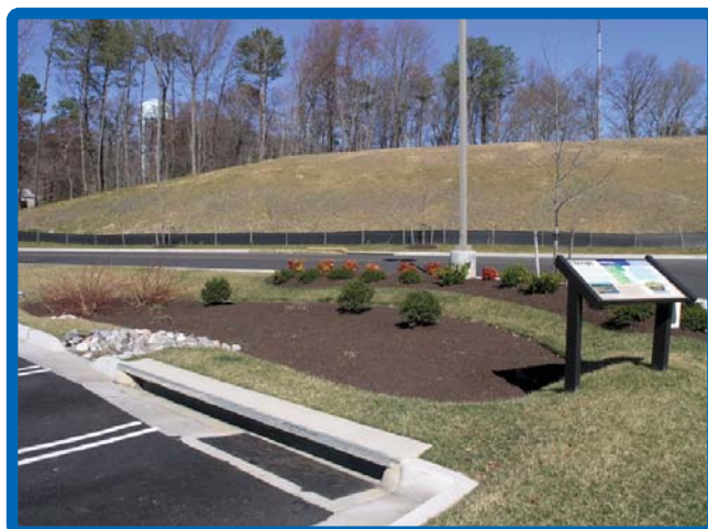
Bioretention area at Ukrop's Supermarket on Forest Avenue, Richmond.
