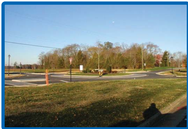
Roundabout at Powhatan County Courthouse.
